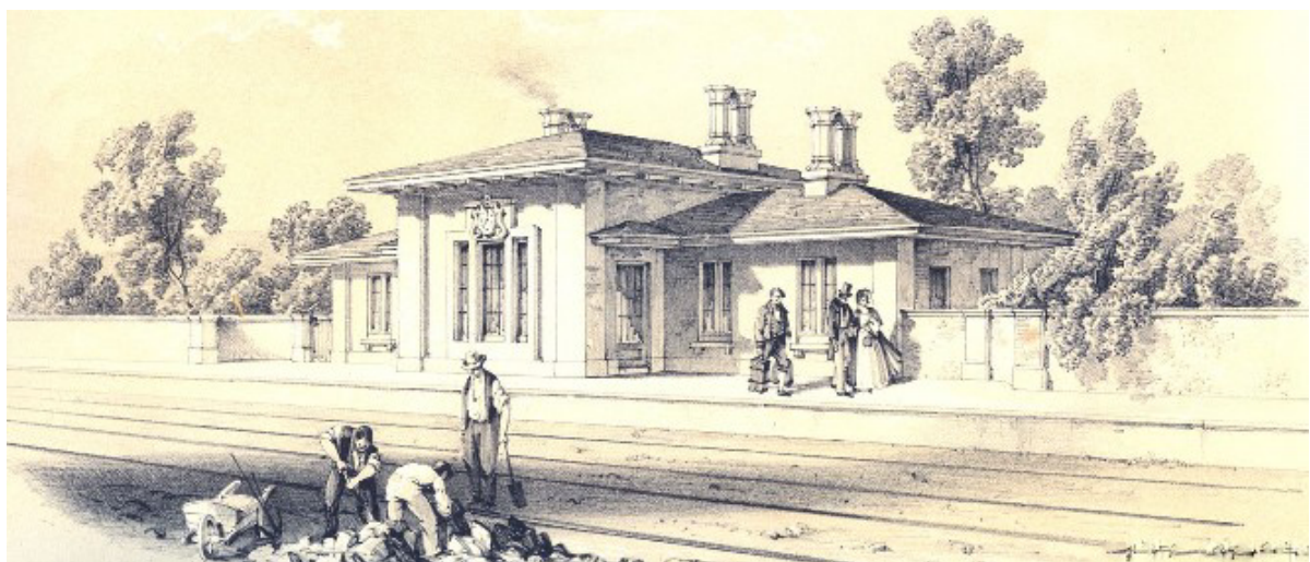
Figure 4. Wingfield station in Derbyshire, designed by Francis Thompson and drawn by Samuel Russell in 1840 when the line was opened. It was closed in 1967; the line however is still open and the building still stands, albeit in very poor condition.
